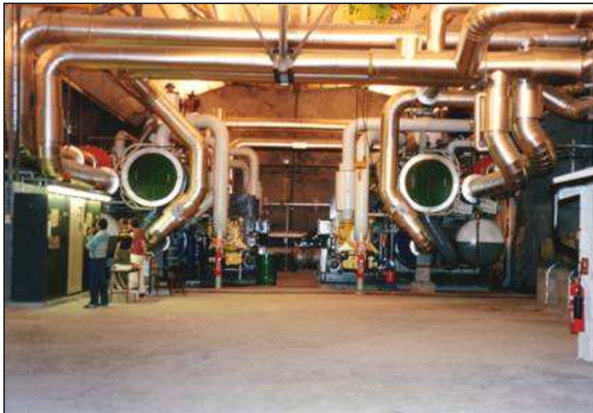
Machine room, 2 Unitop® 28/28 with heat distribution pipe work
