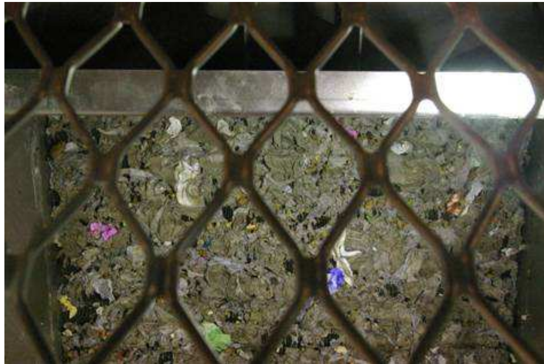
Waste water filter station Mechanical filtration
