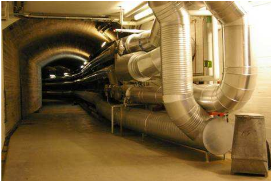
Entrance tunnel, with heat distribution pipe work
