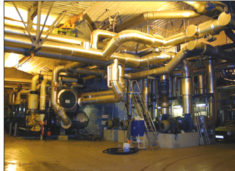
Machine room, left Unitop® 28/28, right: heat/cold distribution pumps
