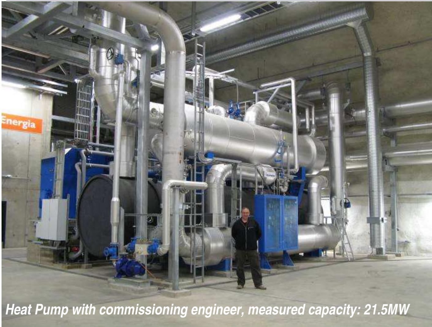
*Heat Pump with commissioning engineer, measured capacity: 21.5MW*
